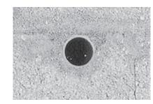
1. After core drilling wall place sleeve in opening and clip-fit external grille.
