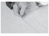
2. Locate position of sleeve internally and apply template of required size.
