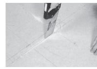
3. Cut out internal lining to required dimension.
