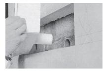
4. Ensure ventilator body and male coupling is in alignment.
